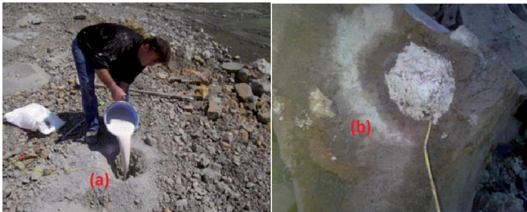
Figure 2.12: (a) Application of plaster paste into the blasthole collar; (b) Blasthole filled with hardened plaster (Cevizci, 2013)
