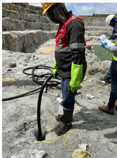
Figure 3.8: Charging explosives (Source: Photo taken on site)
