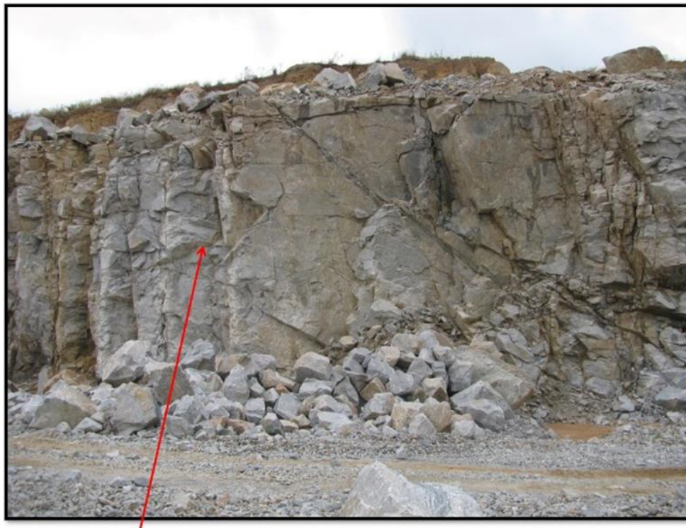
Natural Jointing and Blasting Creates Blocks, East Bench
